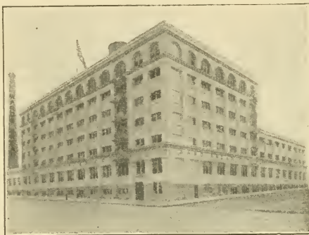
NEW YORK PLANT Southern Boulevard and E. 143rd St., Bronx
